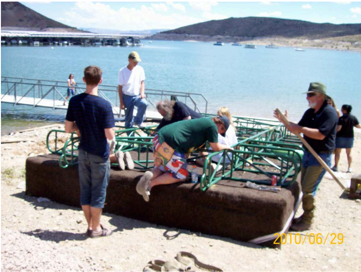
Figure 2. The suspended spawning island provided by Floating Islands West (FIW) provides a structurally sound floating platform with an adjustable suspended mid-section that will be used for aquatic vegetation propagation and experimentation.
