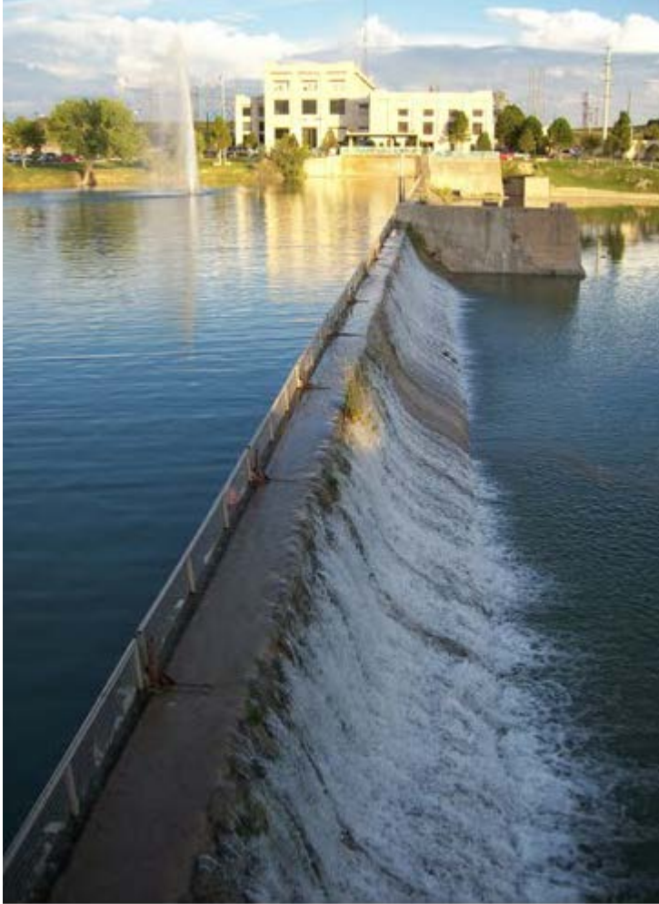
The Carlsbad municipal lakes (Upper and Lower Tansill lakes) are separated by an old dam, allowing for comparative studies between the pools. Photo by Gjorasvik, Date unknown.
